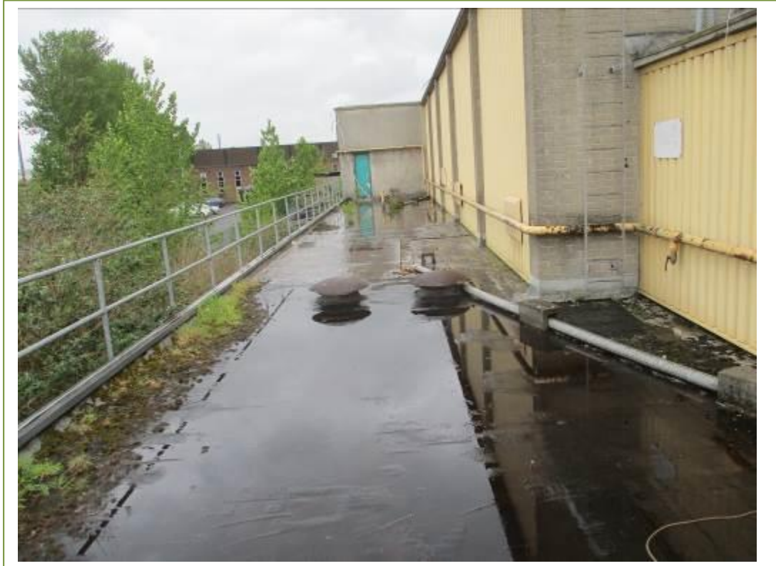
Metal side cladding. No Asbestos Containing Materials (ACM's) detected
