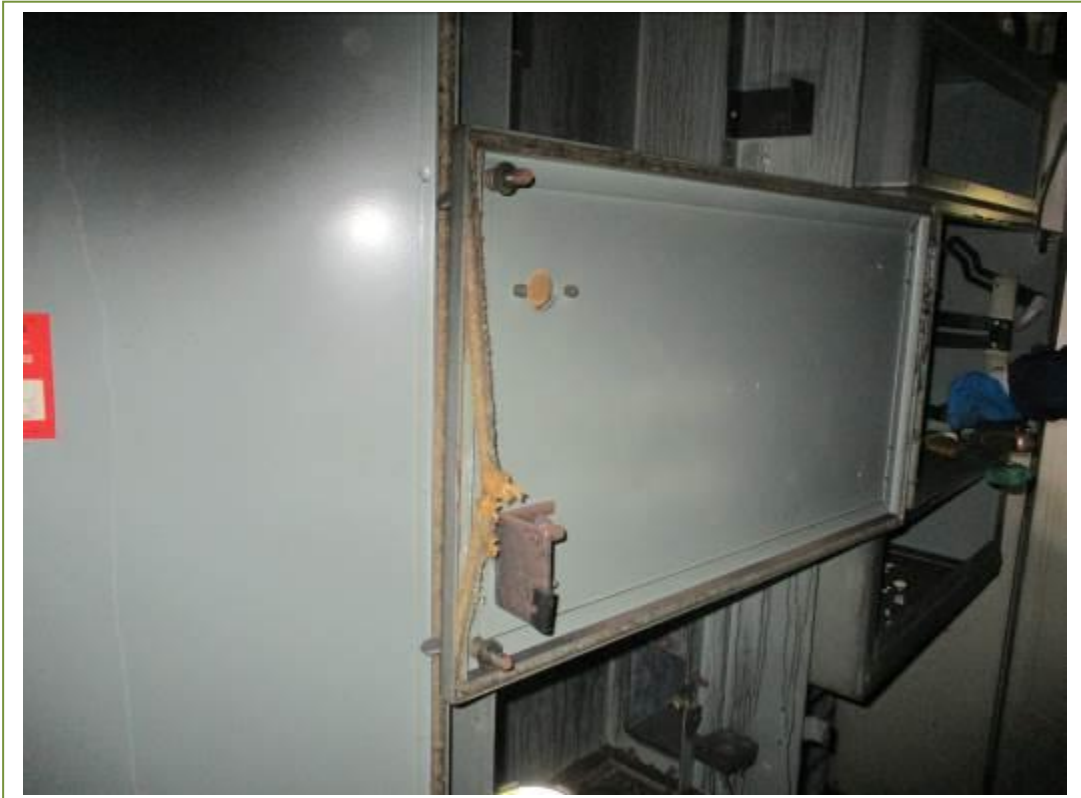
Rope on modern electrical box doors in block 1. No ACM's detected
