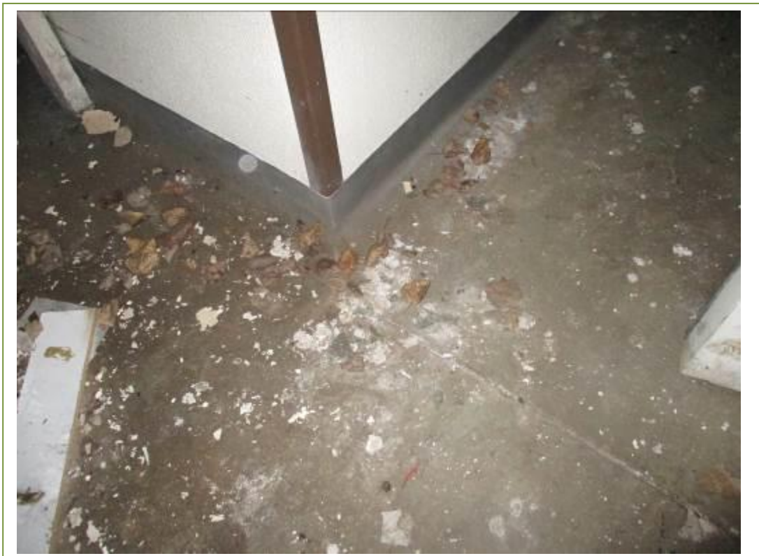
Thermal insulation debris can be seen throughout the floor of the kitchen area
