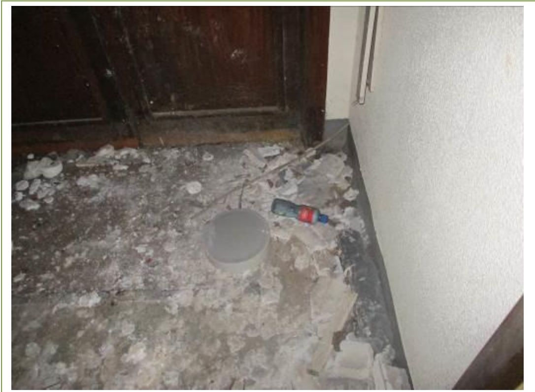
Damaged thermal insulation directly under the pipework
