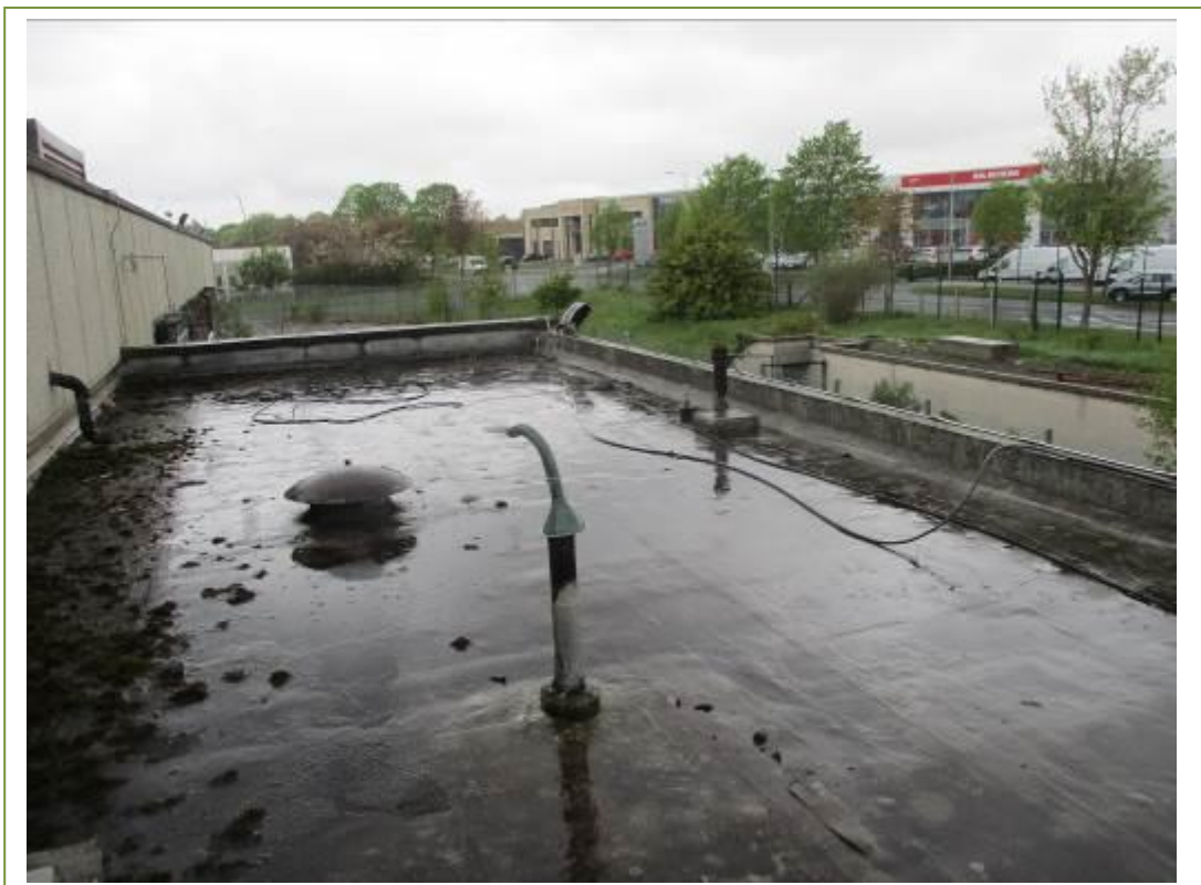
The felt on the lower flat roof to the front had the same felt applied
