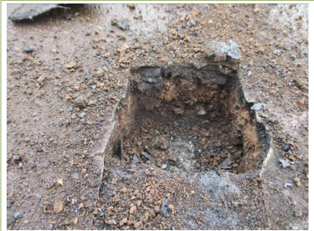
Closer view of the asbestos containing felt
