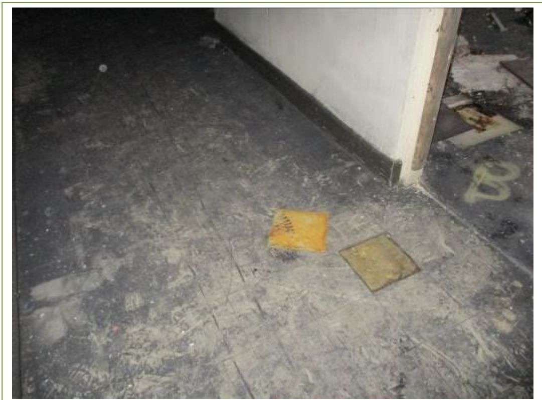
Floor tiles and evostick adhesive. No ACM's detected
